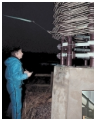
Above: Stellan Nilsson, head of SAQ, finds a melted wire on one of the aerial coils during a test transmission.
