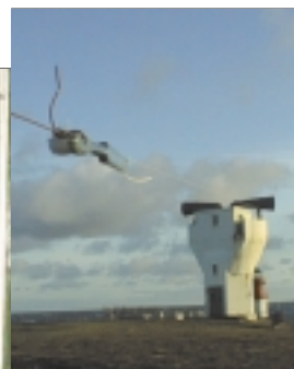
Toothbrush insulator at the end of the 200m-long antenna.
