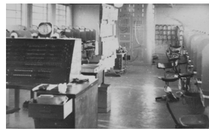
Another view of the Hanslope Park intercept station, showing at the far end the massive construction of the set of wideband amplifiers, but with the original 'concentrator' torn out.
