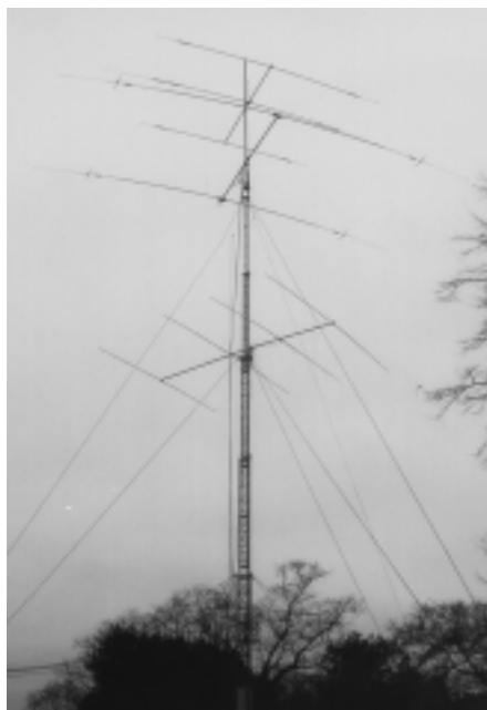
One of the 70ft towers, supporting HF beams.
